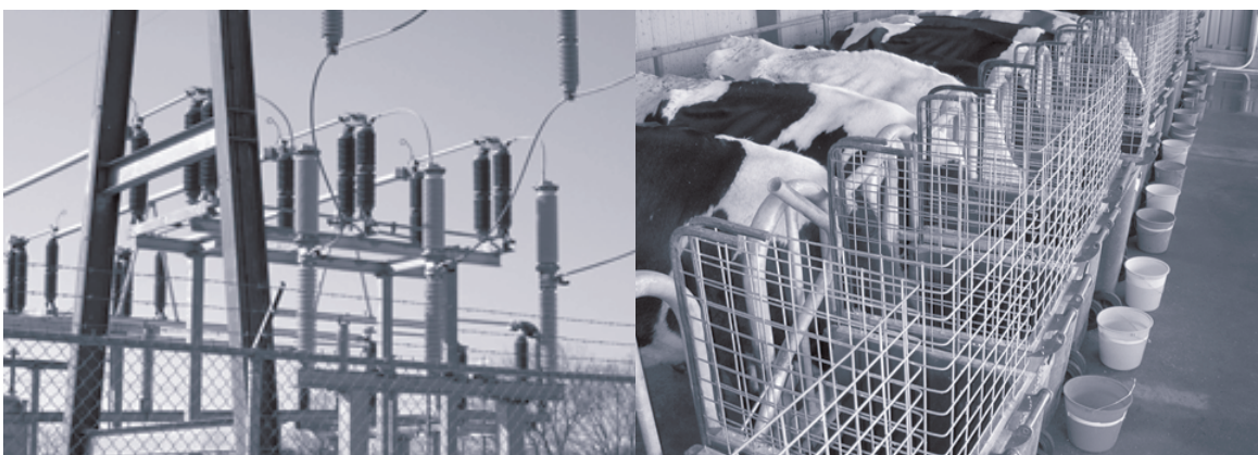
> Electricity substation insulators.
